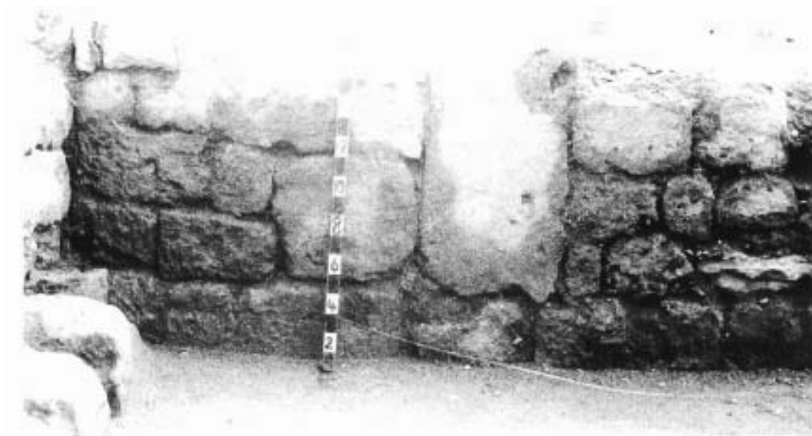
Figure 6. Orthostatic construction in south wall of Building A, Courtyard I.
